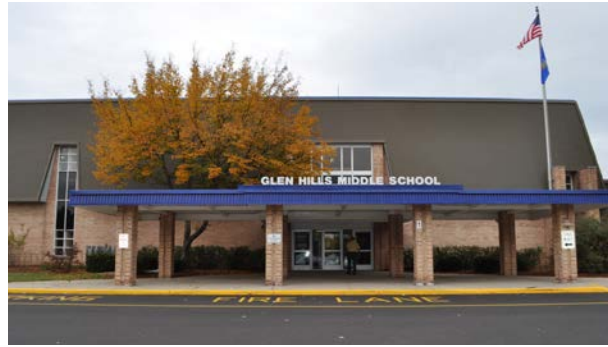
Glen Hills Middle School – Glendale, Wis. Certified LEED Platinum in 2012
